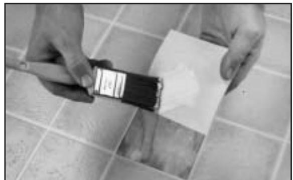
**Fig. 6.** Apply a thin coat of adhesive.
