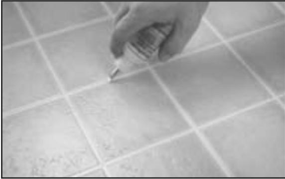
**Fig. 7.** Seal seams with the recommended seam sealer.
